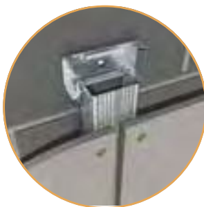
155 Furring Channel Fixed to Wall
