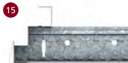
■ INTRODUCING TRIM TO THE SUPPORT CLIPS
